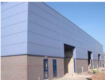
Twyford Road units nearing completion
